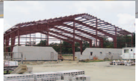
At Orrville High School's new multipurpose facility, the pre-engineered metal building has been erected and masonry work has started.
