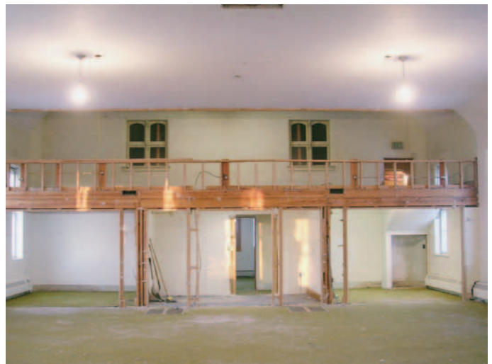
A "before" picture of the sanctuary just after demolition had begun.
